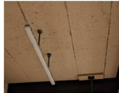
Example of RAAC in flat roofs and floors
